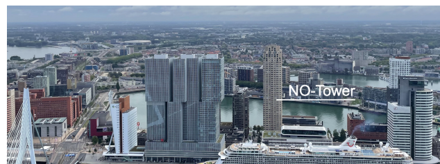
Figure 1. NO-Tower and surrounding in Rotterdam
